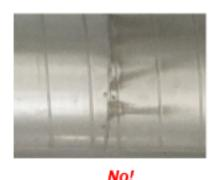
Better Appearance --- Exposed duct systems have to be sealed too. And no one wants the sight of field-applied mastic covering each duct joint. With Gasket-Tite, the sealant is integral to the joint --- and on the inside. Do you ever see those ugly dust streaks at the joints of exposed duct systems? That's the sign of an unsealed or poorly sealed duct joint. The Gasket-Tite system gives you a full and consistent seal at all 360 degrees of the joint circumference.
